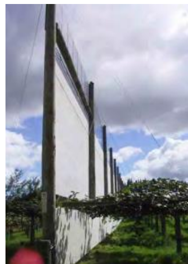
Figure 17: Artificial wind breaks provides instant shelter and maximizes the productive land area. Sourced from NZKGI Kiwifruit Book 2019.
